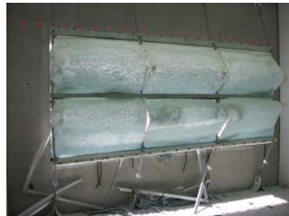
ABOVE: Pre-drilled SGP laminated glass panels attached to horizontal steel tube members and supported by steel rods. The rods were then mechanically anchored to steel plate clips at floor and ceiling.
