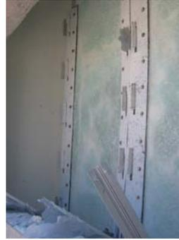
ABOVE: Pre-drilled SGP laminated glass sheets attached to steel frame members to make individual panel frames. These frames are then mounted on clips fabricated from steel channel section which were welded to steel tube supports
